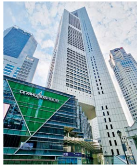
OUB Centre (Singapore) Modernization/Completed The building constructed as the tallest building in Asia in 1986. There are 19 elevators installed.
